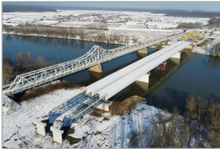
Figure 5: Launching of Bridge Structure
