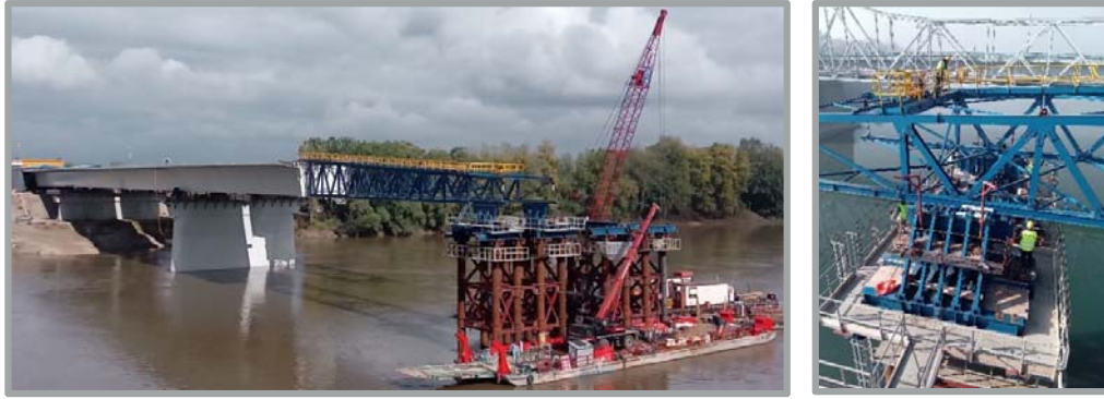
Figure 14: Temporary Pier D01
